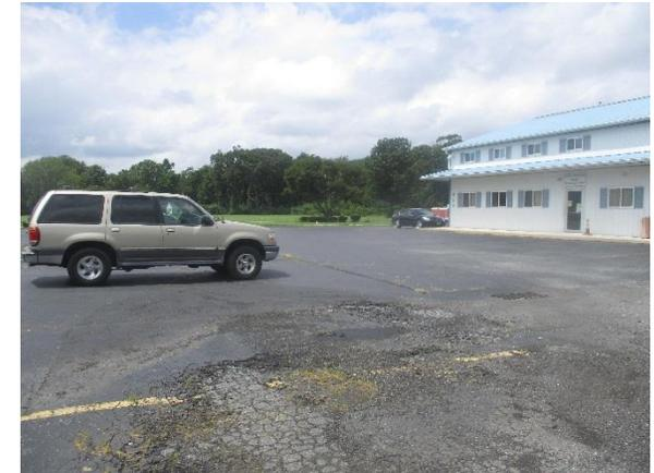
Stormwater is currently directed to existing catch basins. The main parking lot is in poor shape, and parking spots can be replaced with porous asphalt to capture and infiltrate stormwater runoff. A preliminary soil assessment suggests that the soils have suitable drainage characteristics for green infrastructure.
