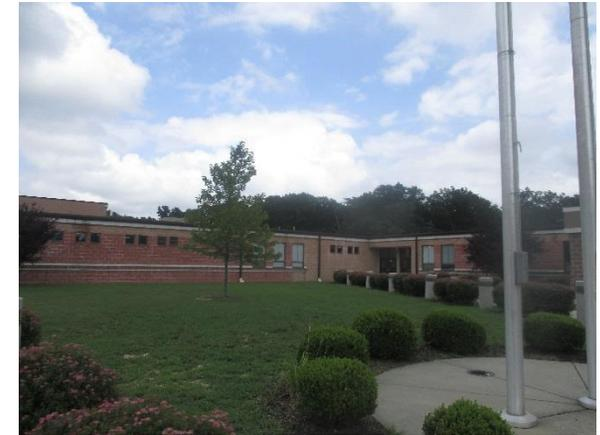
Stormwater currently drains from disconnected downspouts. A rain garden in between the two main entrances of the school can capture, treat, and infiltrate roof runoff as well as add to the existing landscaping of the school. A preliminary soil assessment suggests that the soils have suitable drainage characteristics for green infrastructure.
