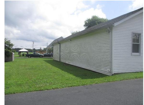
Stormwater currently drains to the roadway. Installing a rain garden adjacent to the building can capture, treat, and infiltrate roof runoff. A preliminary soil assessment suggests that the soils have suitable drainage characteristics for green infrastructure.
