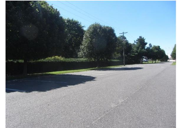
Stormwater is currently directed to existing catch basins throughout the parking lot. Parking spots on the far east and west sides of the parking lot can be replaced with porous asphalt to capture and infiltrate stormwater. A preliminary soil assessment suggests that the soils have suitable drainage characteristics for green infrastructure.
