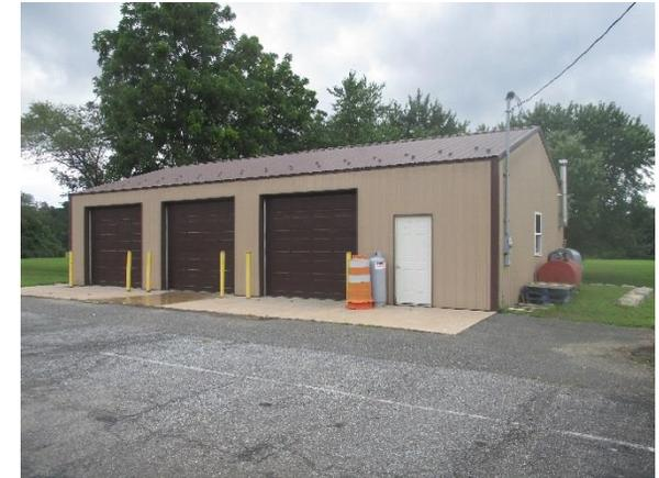
Stormwater currently drains from the property and the roofs of the buildings without downspouts. A cistern, as well as a downspout, can be installed on the northwest corner of the west building to capture stormwater runoff. The water can then be used for washing vehicles or for other non-potable uses such as car wash fundraisers or watering existing landscape plants. A preliminary soil assessment suggests that the soils have suitable drainage characteristics for green infrastructure.
